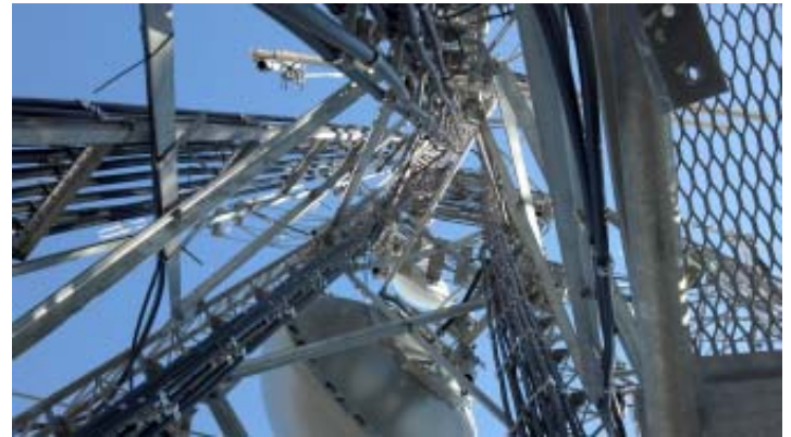
Looking up the middle of the Mt. Ord tower.
