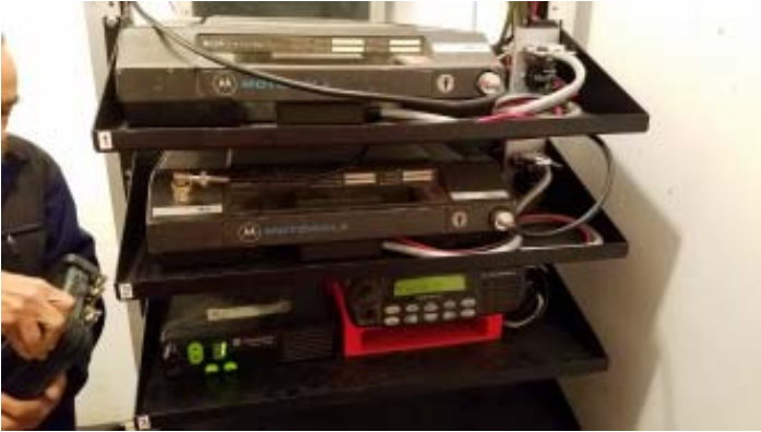
Motorola Micor radios used for the control and VHF repeater with Motorola CDM radios below for the UHF repeater.
