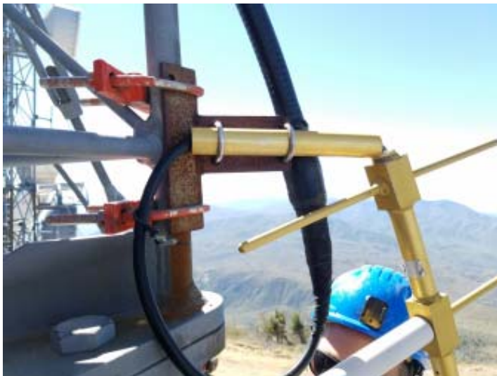
Mt. Ord link antenna to Shaw Butte didn't survive a falling ice hit.
