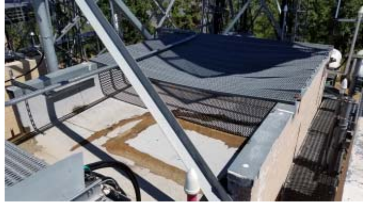
Mt. Ord building roof showing the temporary patch and bent ice guard.
